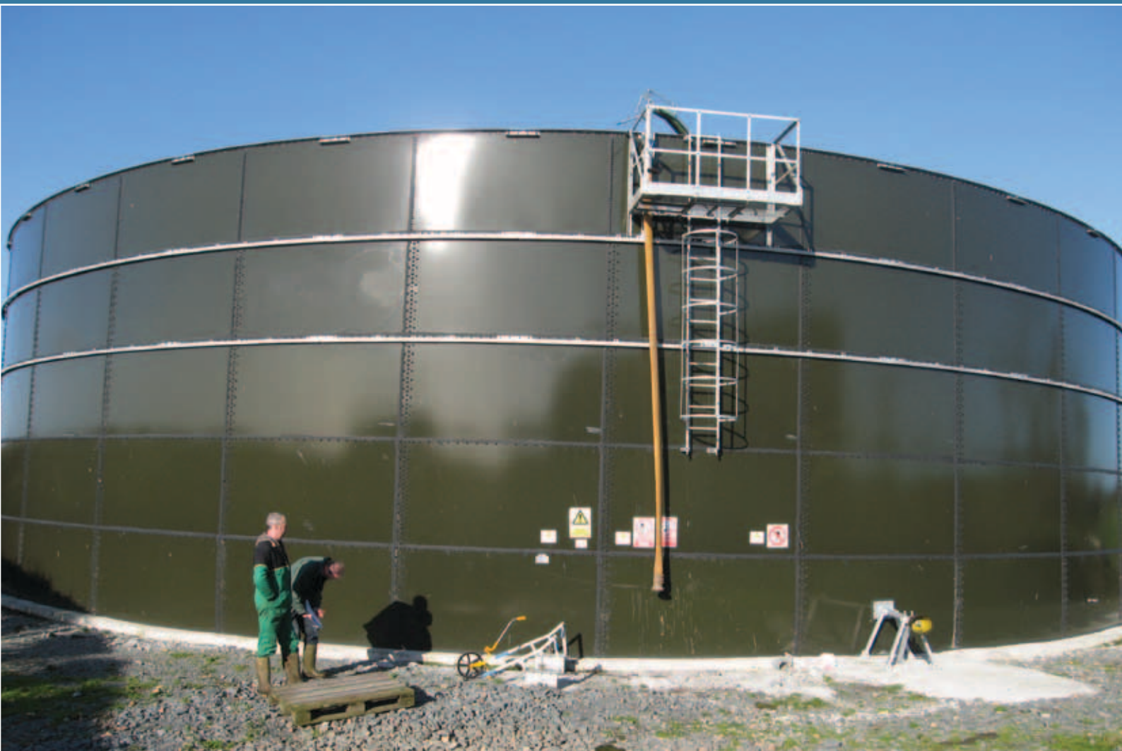
An above ground steel slurry tank, under construction.
