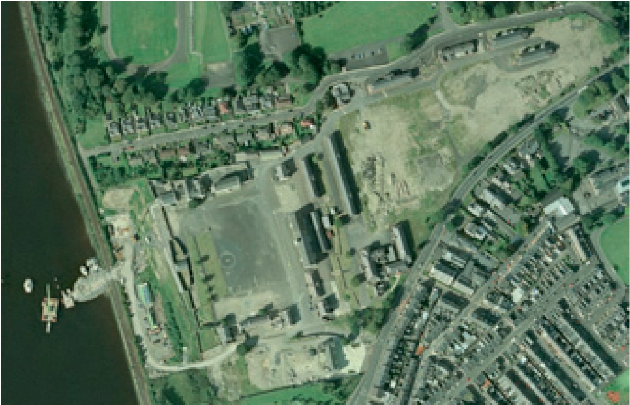
Aerial view of the Ebrington site: OSNI
