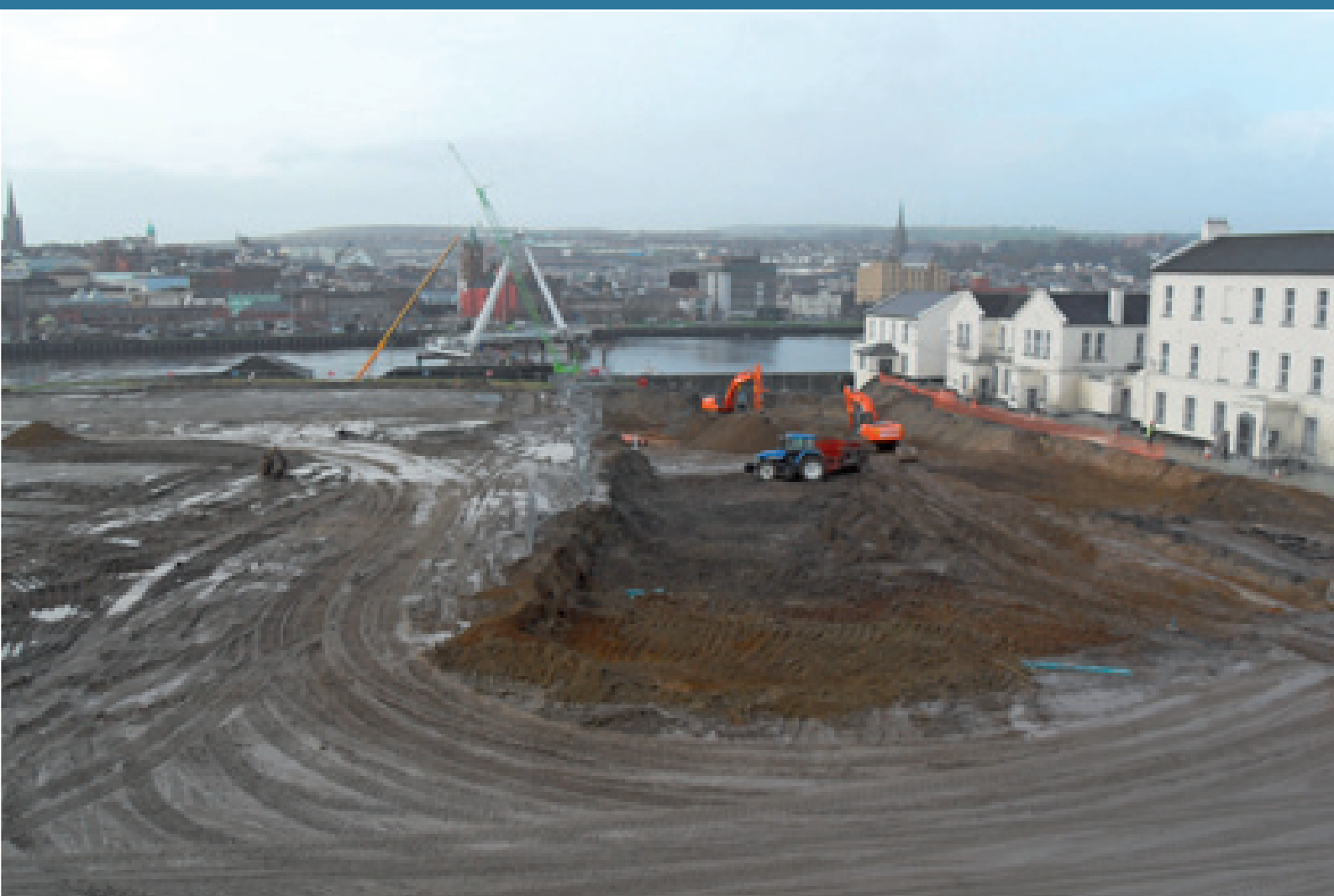
Construction work underway at Ebrington Barracks Site. Photo courtesy of Ilex
